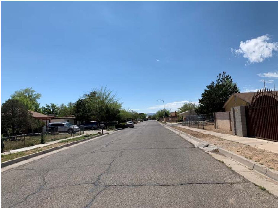
Figure 3: Gwin Road looking east
